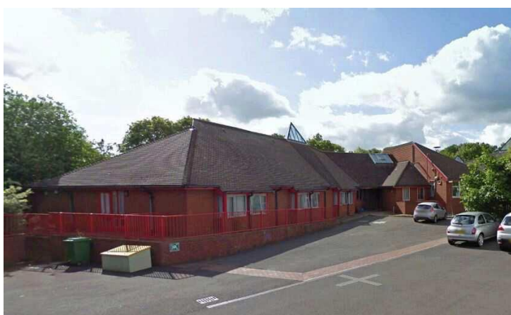
Bennett House, Park Lane, Woodside, Telford
